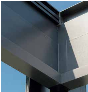
Water run-off built into support
